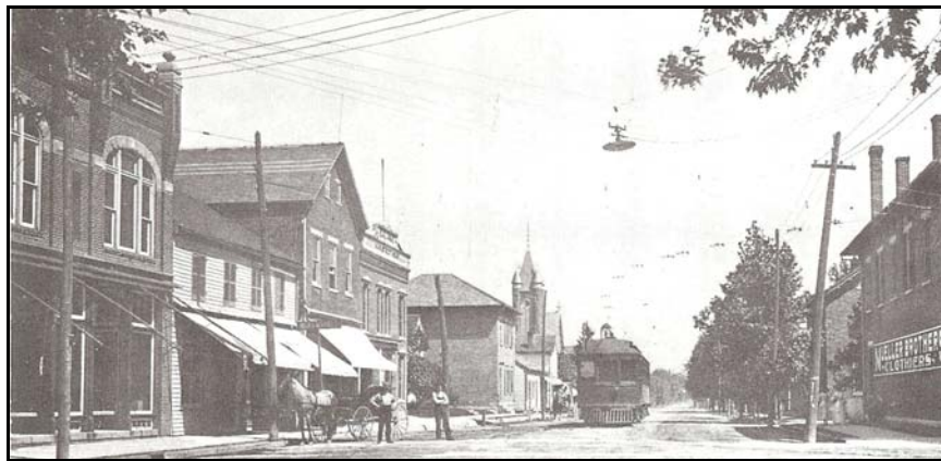
NORTH MAIN ST. IN NEW BREMEN – LOOKING NORTH
