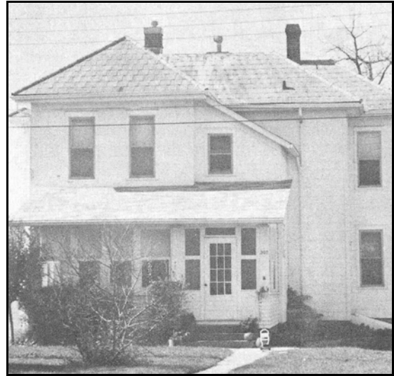
St. Peter's Church parsonage (October 1991)
