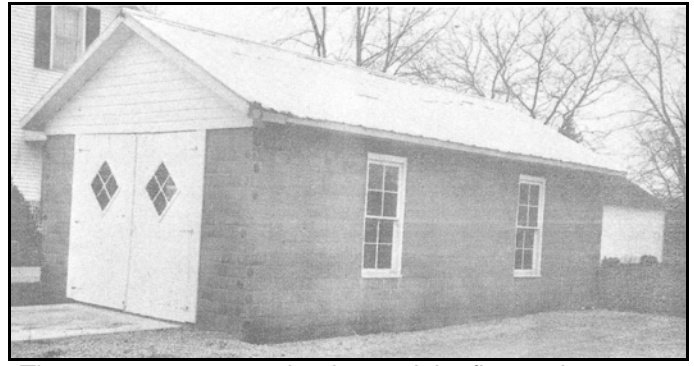
The cement structure that housed the fire engine at one time still stands in Lock Two today – June 1992.
