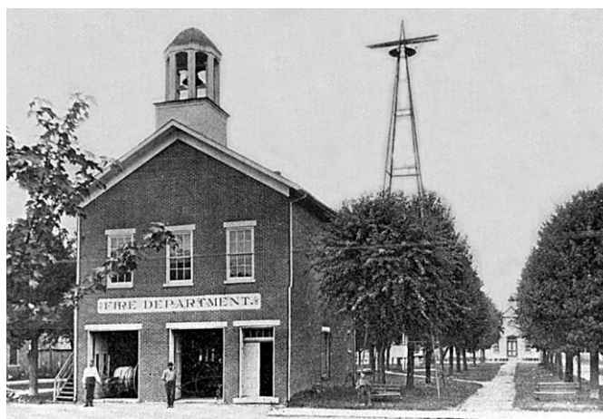
Northern Fire Company (111 N. Main Street) established 1857 and Town Hall.
